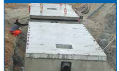
Terreinafwatering asfalt Rotterdam
