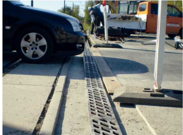
HYDROblock, Project: Spoorwegovergang, Frankfurt/Oder
